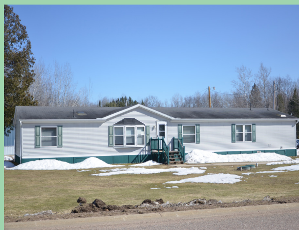
Legal Building Closed
