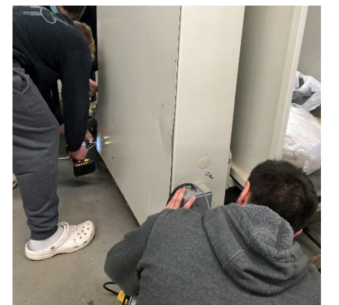
Checking wiring & function of the elevator
