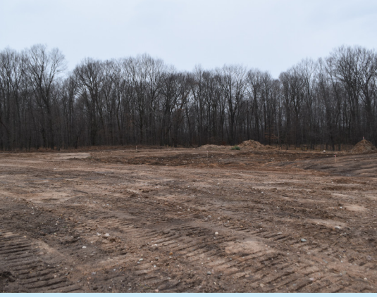
November 2022 ground breaking started
