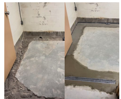
French Drain Install
